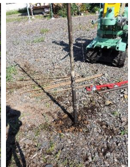
Set in borehole
